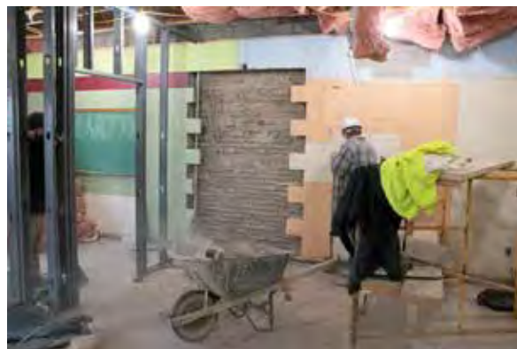
The renovation of Martin Hall begins.
